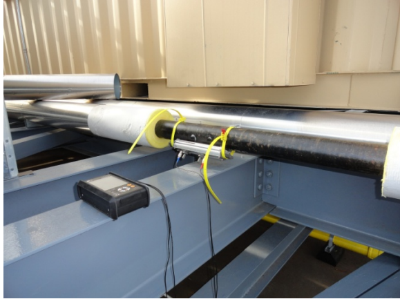
Ultrasonic Flowmeter Verification of FL2
