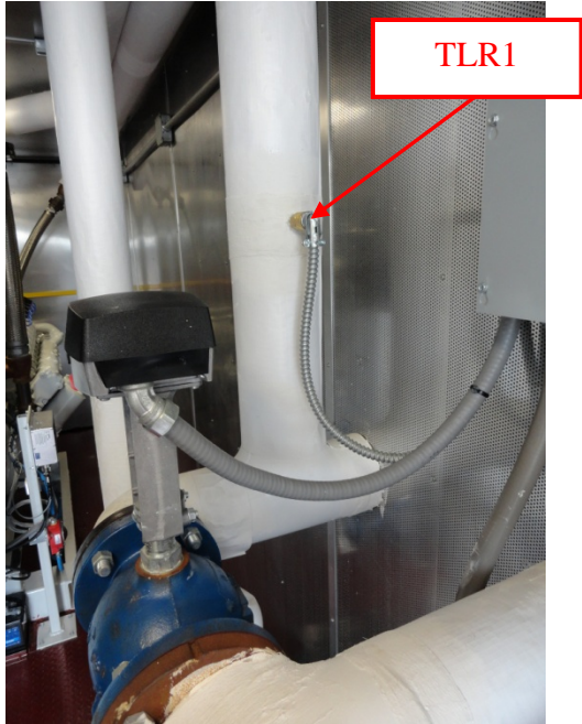
Primary Loop Return Temperature (To CHP)
