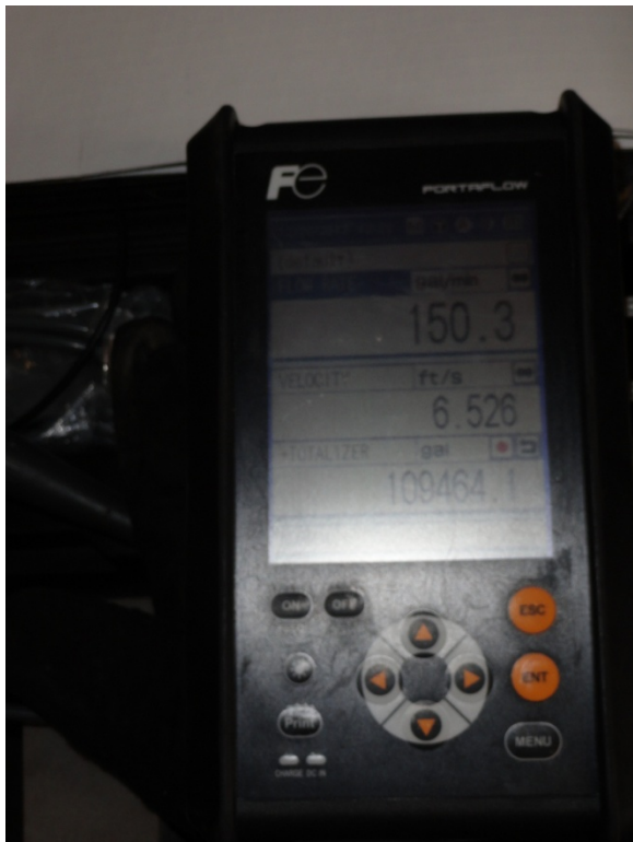
FL1 Flowmeter Reading (Typ of FL2 also)
