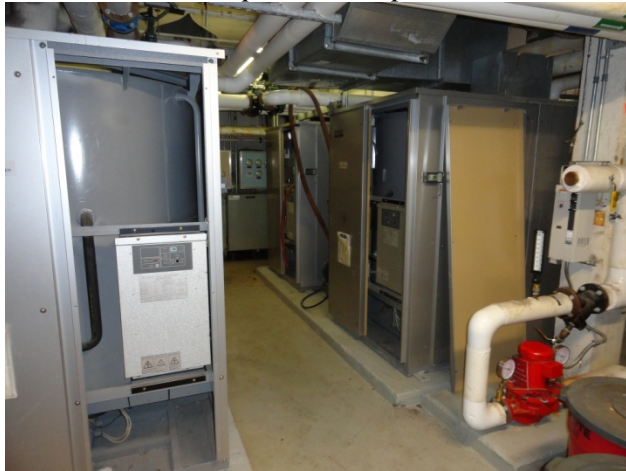
Absorption Chillers (1 of 3 typ)
