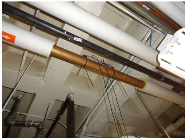
PortaFlow Ultrasonic Transducer
