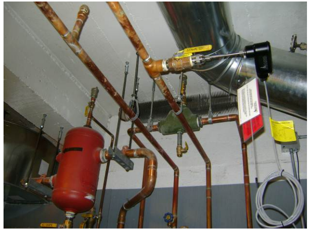
Boiler Loop -Onicon F-1111 flowmeter.
