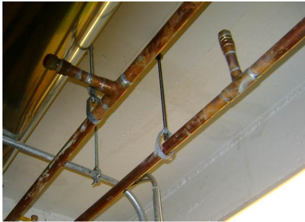
Boiler Loop - thermowells.
