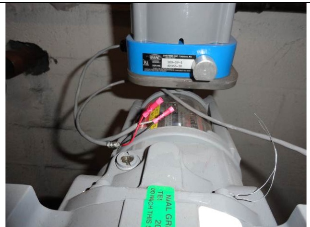
Natural gas meter wiring
