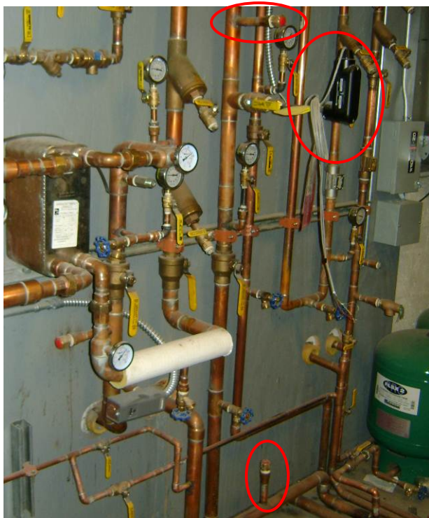
Boiler Loop - thermowells.
