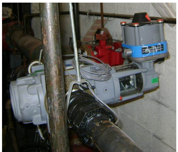
Boiler Loop -Onicon F-1111 flowmeter.
