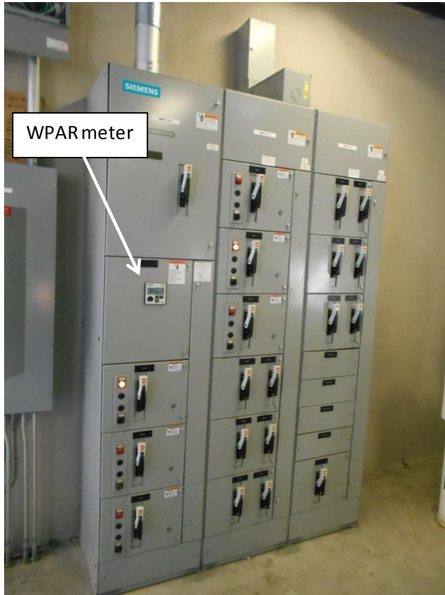
Figure 4. MCC-1 Containing CHP Parasitic and Non-parasitic Loads
