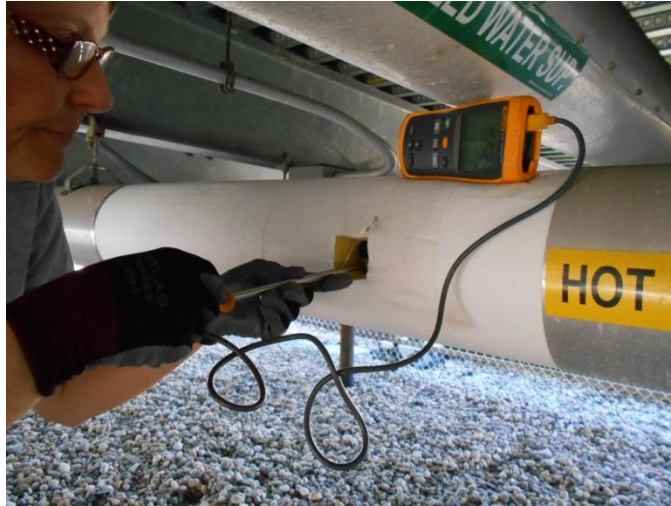
Pipe surface measurement
