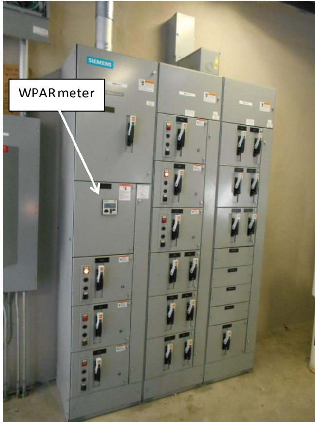
Figure 2. MCC-1 Containing CHP Parasitic and Non-parasitic Loads
