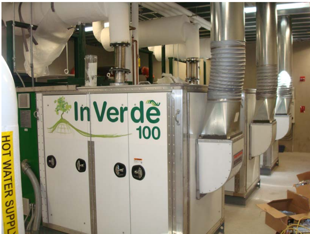
Figure 1. Photo of Engines installed in Roof-top Mechanical Room
