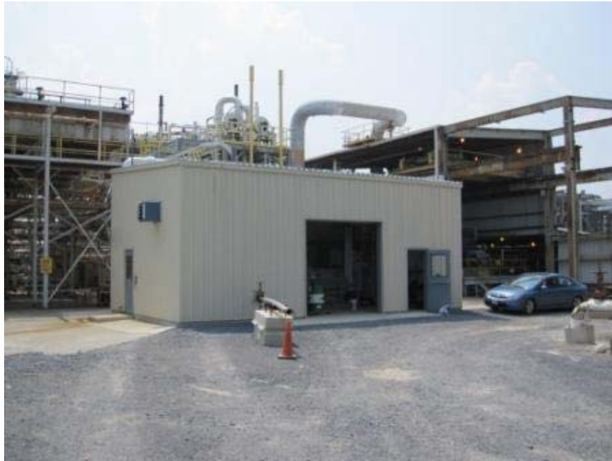
Fig 2: New Steam Turbine Generator Building
