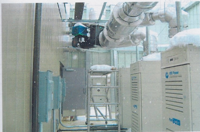
Figure 1. Microturbines during installation
