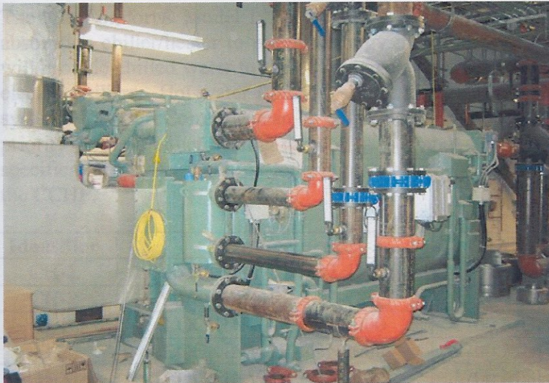
Figure 2. Absorption Chiller during installation
