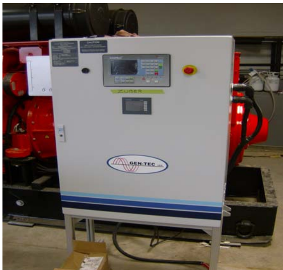
Gen-Tec engine control panel
