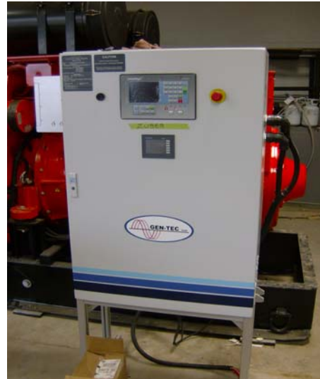
GenTec Panel with power output display
