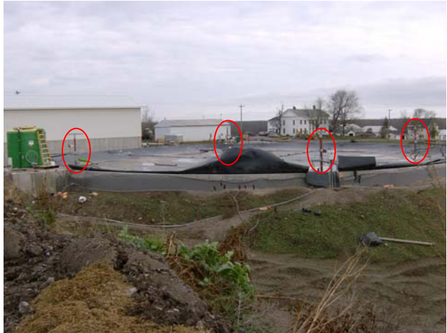
Digester and 4x mixers
