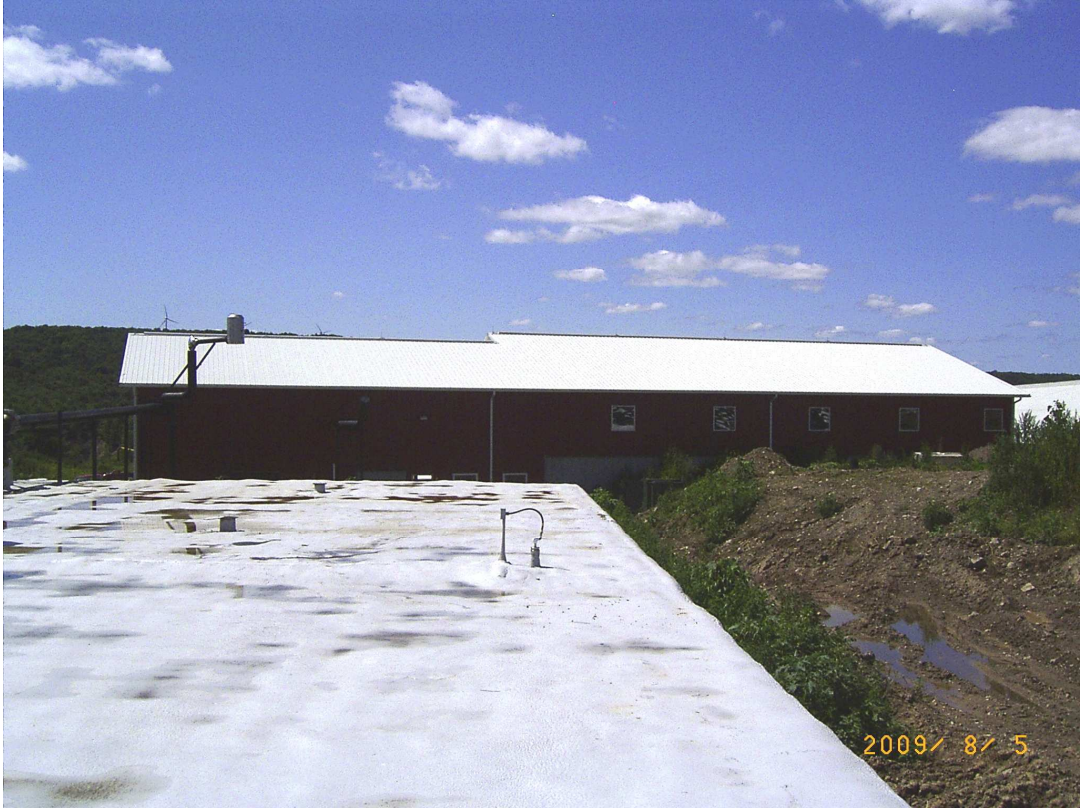
Foreground: Top of Digester, Background: Engine Room and Solids Building
