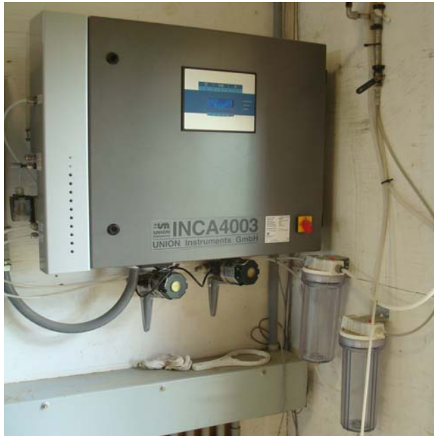
INCA 4003 gas analyzer and sampling solenoids (left H 2 S into scrubber, right H 2 S out of scrubber).
