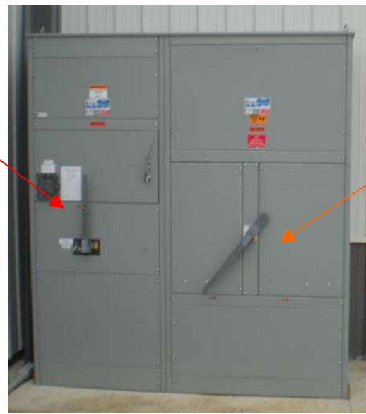
800 Amp GFI Breaker/Transfer Switch
