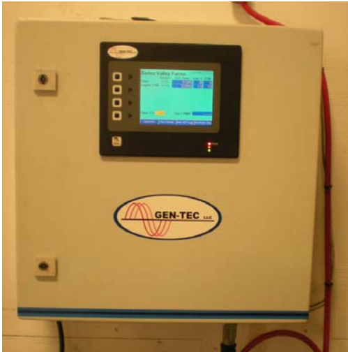
Gen-Tec/Red Lion Data Logger, kWh and mass flow display
