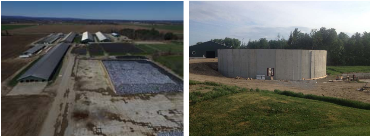
Figure 1: Aerial View of Adirondack Farm LLC (left) and Digester Construction Progress (right)
