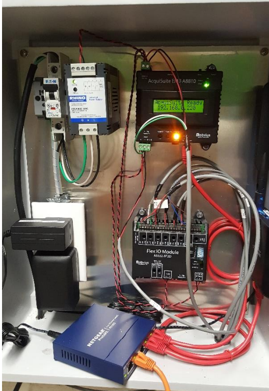
CDH M&V enclosure with Cradlepoint cellular modem mounted on right side of enclosure
