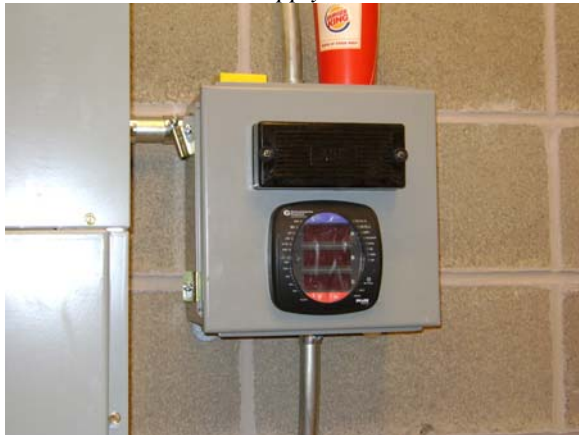
Shark 100 Power Transducer For Combined Microturbine Power
