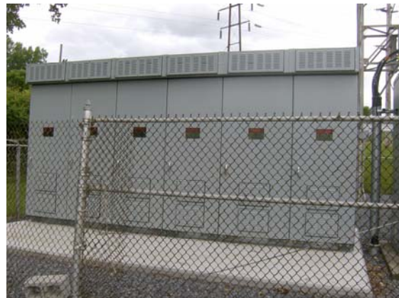
13,000 panel - location of CT's measuring engine output
