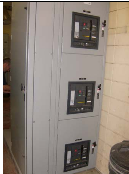
Breakers - Generators 1 & 2, and feeder to facility.
