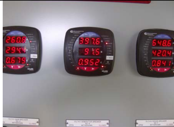
Power displays (left to right) - kW purchased from utility, kW generated (both generators), total facility demand.
