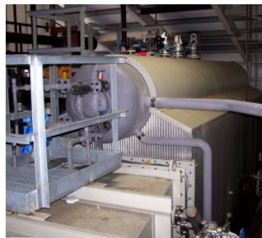
FIGURE TYPICAL HEAT RECOVERY STEAM GENERATOR
