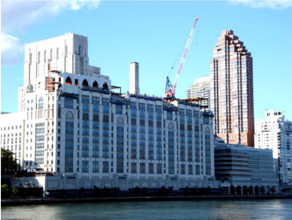
FIGURE NEW YORK PRESBYTERIAN HOSPITAL
