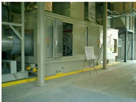
FIGURE TYPICAL PACKAGE GAS TURBINE INSTALLATION
