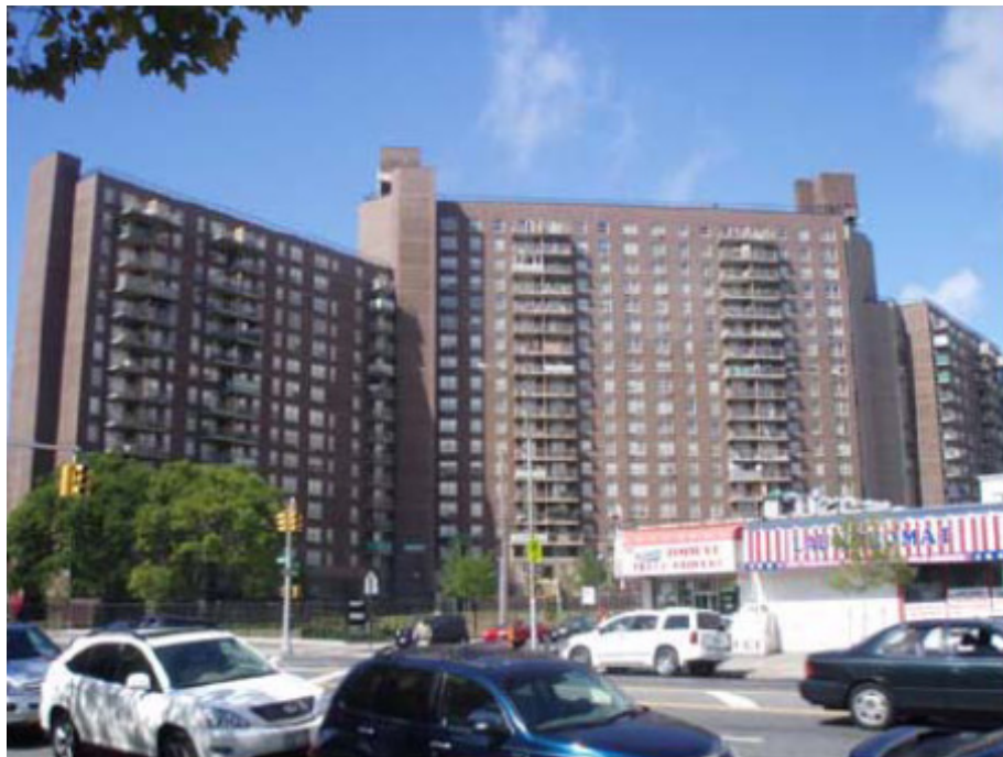
FIGURE 2 SEA PARK WEST IS AN AFFORDABLE HOUSING COMPLEX
