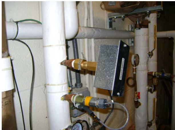
THR1 – on HX wall, right most and top most temp sensor.
