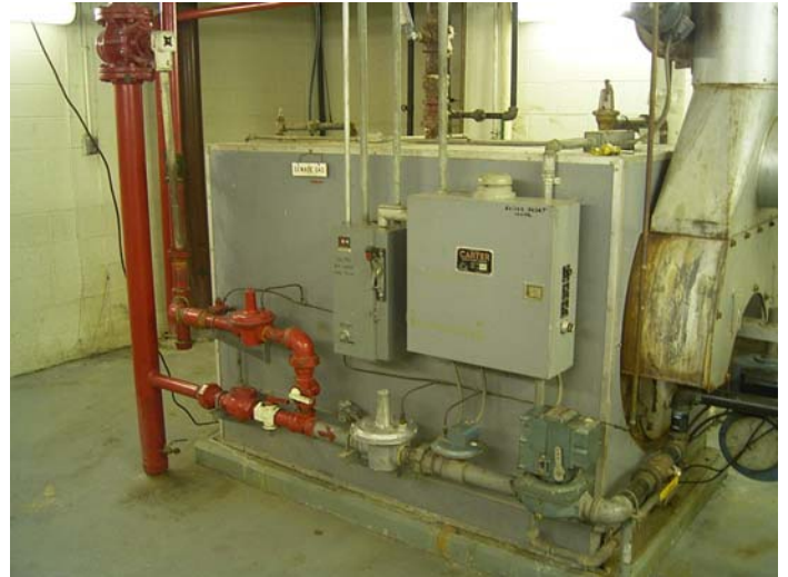
Digester Boiler
