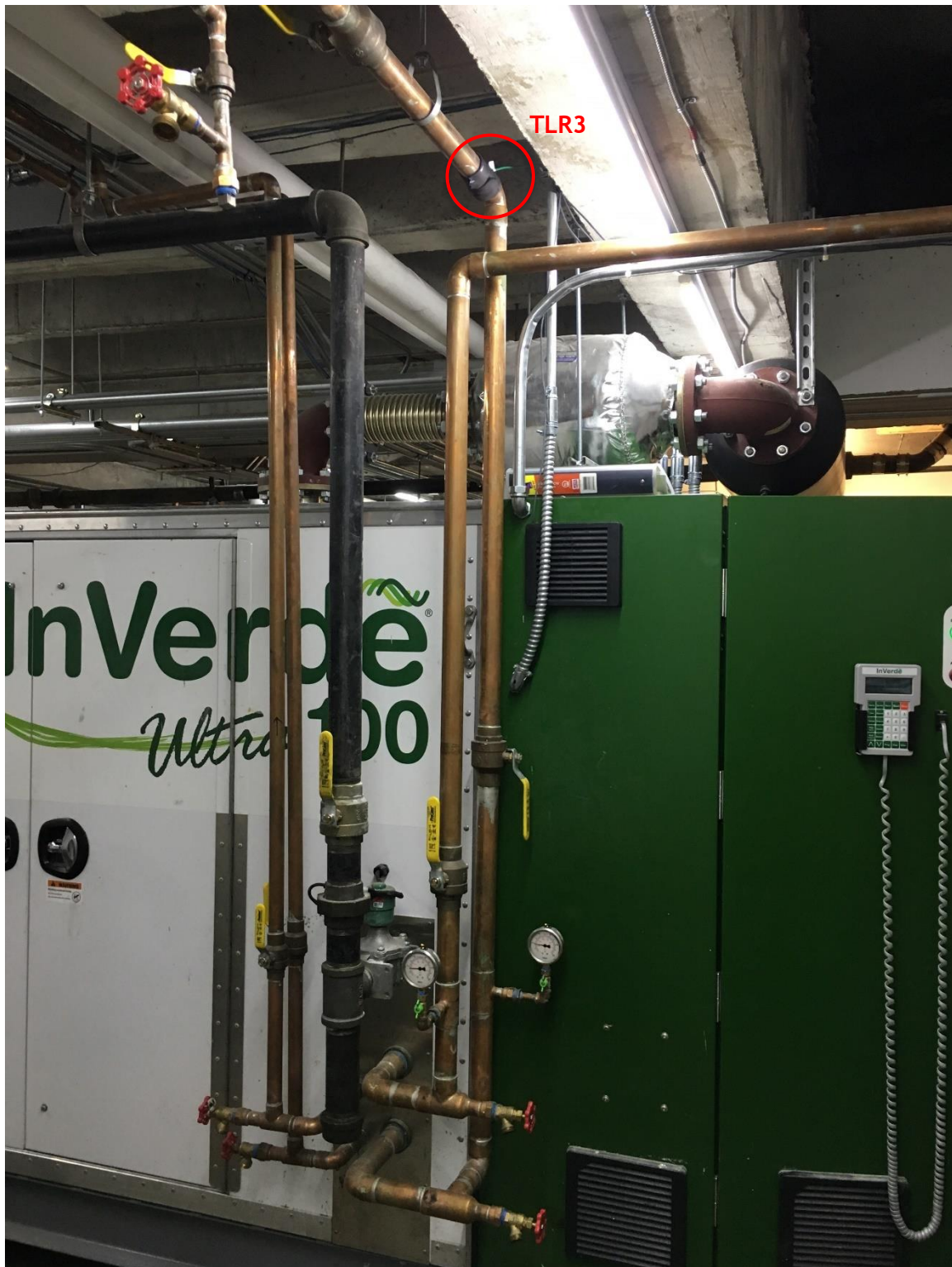
Heat Recovery Supply and Return and Gas Supply on Cogen Unit with TLR3 shown (before gas sub meter installed).
