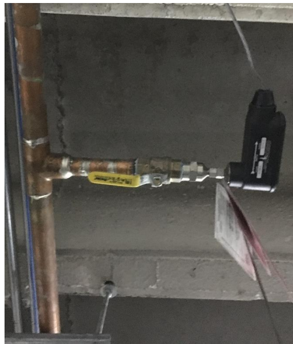
HW Loop Onicon Flow Meter (In Garage)
