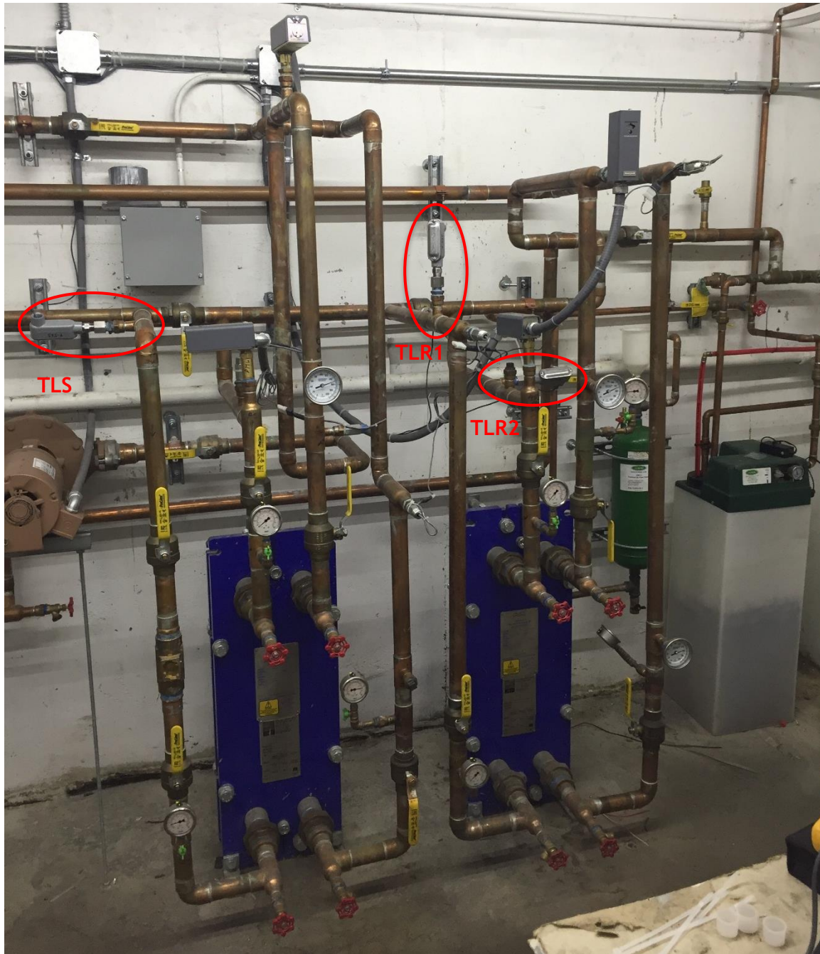
DHW HX (HX1) Left and Condensate HX (HX2) Right with TLS, TLR1 and TLR2 shown.
