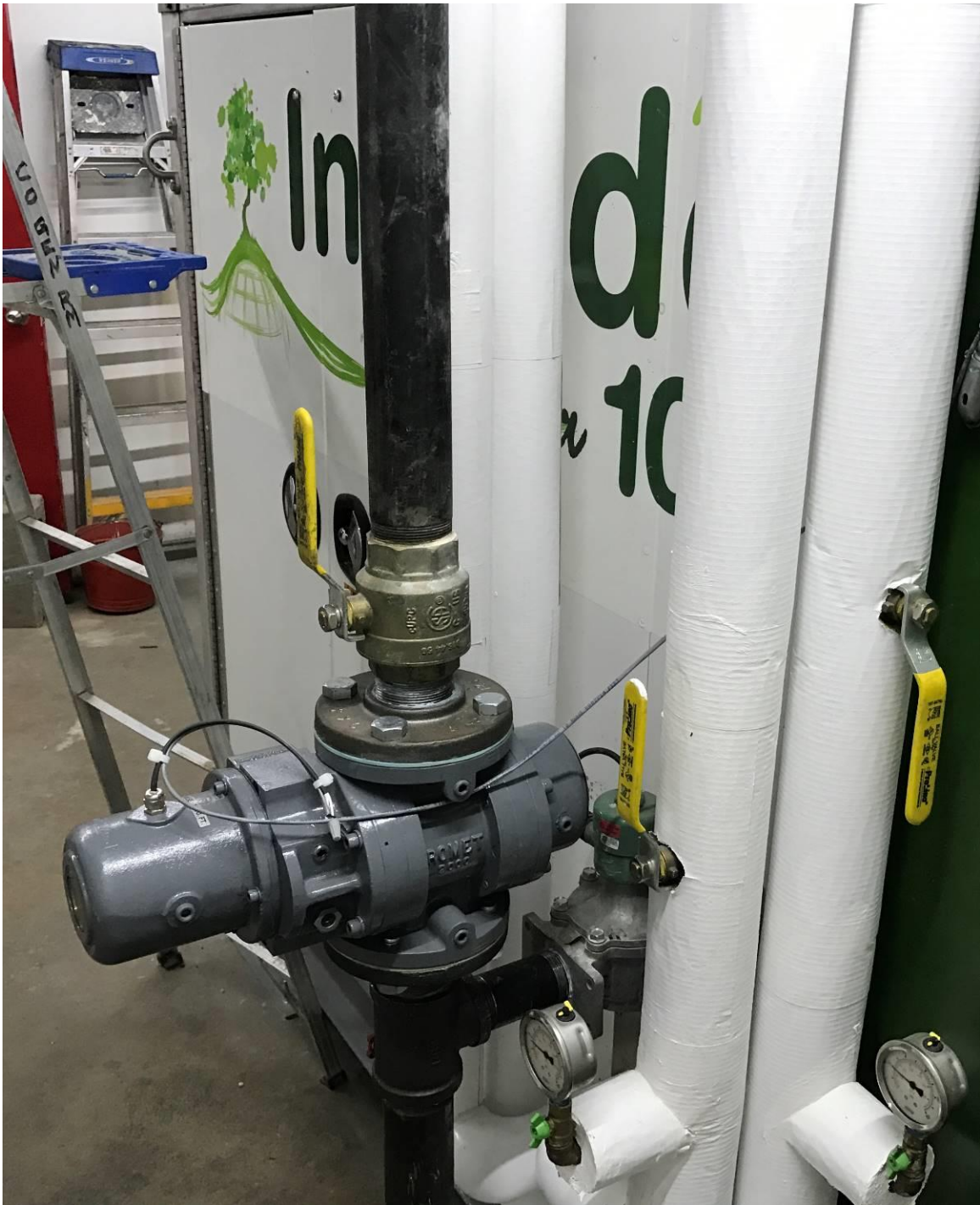
Romet 2000 gas sub meter w/ 10cf/pulse pulser
