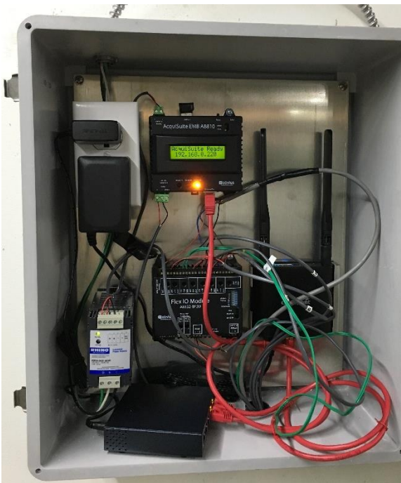
CDH Monitoring Enclosure w/ Obvius Data Logger
