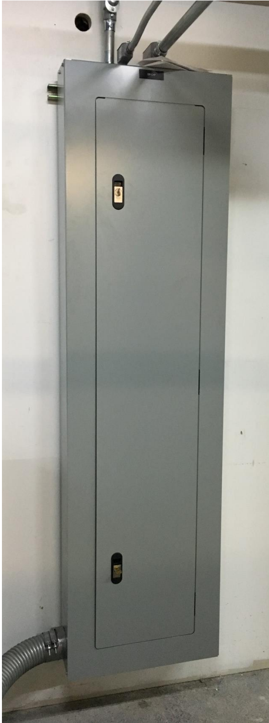
208V Parasitic Panel in Cogen Room
