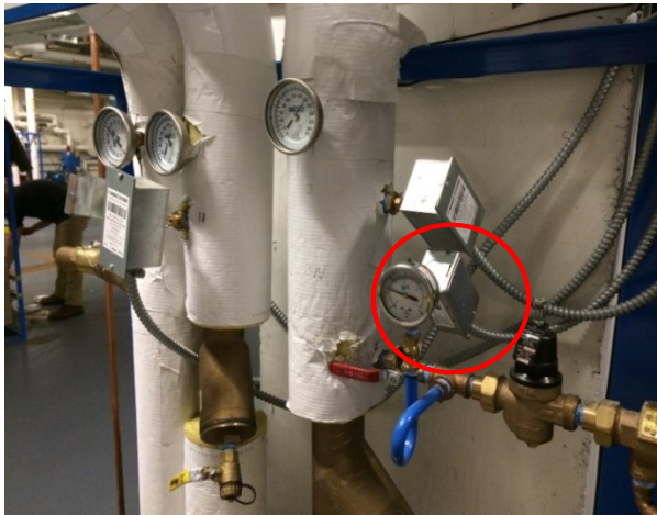
Veris 10k Type II Thermistor (THW1) located on HX1
