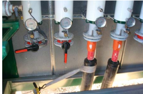
Heat recovery piping; 3x sets of supply and return piping. One set currently used for digester heating, other two sets are spares for future expansion.
