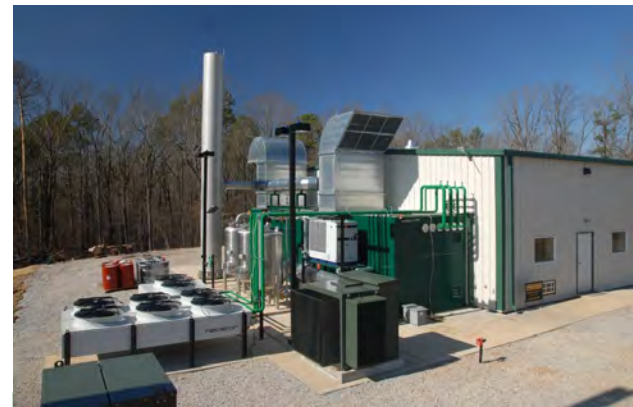
Landfill Gas (LFG) Power Generation Plant with “Plug & Play” Container Module, including Gas Conditioning & Treatment System.
