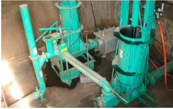
Manure pumps, supply to digester or slurry storage tank.
