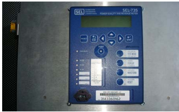
Revenue grade SEL-753 generator power meter.
