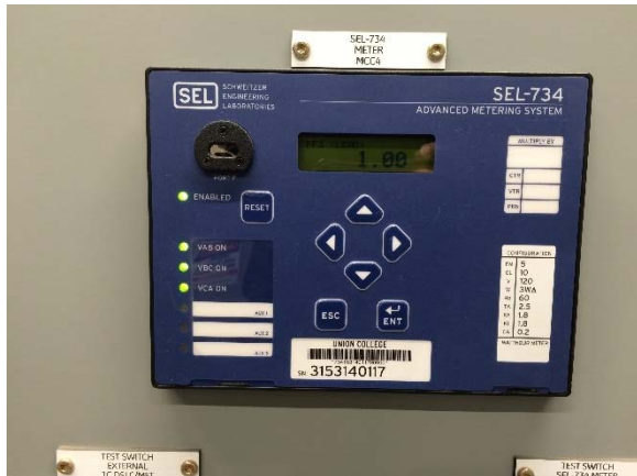
MCC4 Parasitic Load Meter - Typ. (WP3)
