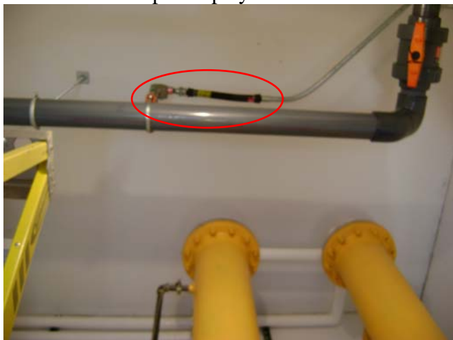
Sage Flow Meter (FG1) – total biogas flow
