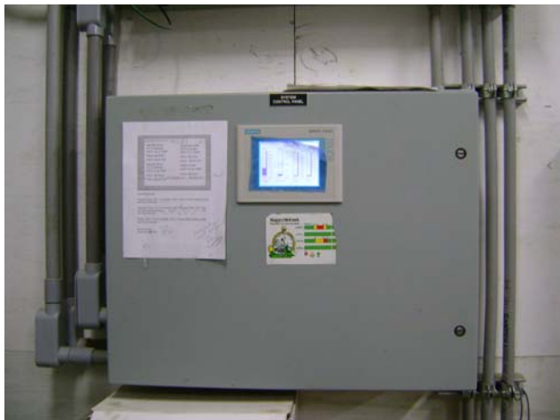
Siemens control panel with Veris Power Transducer's output displayed on far left.
