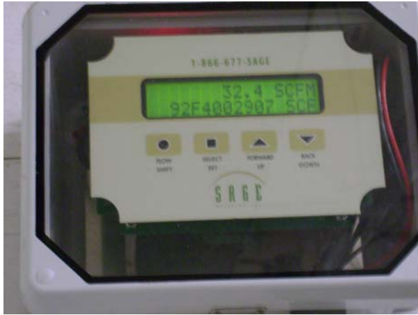
Sage Display (FG1) – total biogas flow
