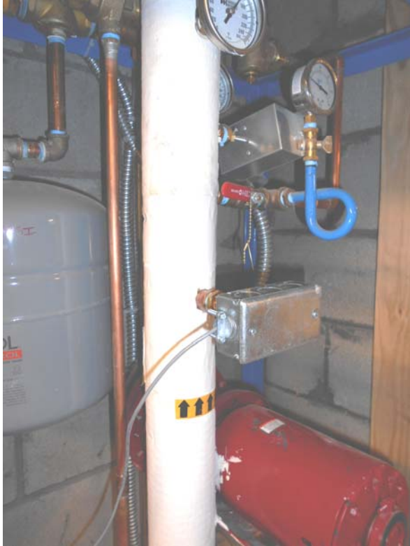
Veris 10k Type II sensors leaving dump HX (THW3)
