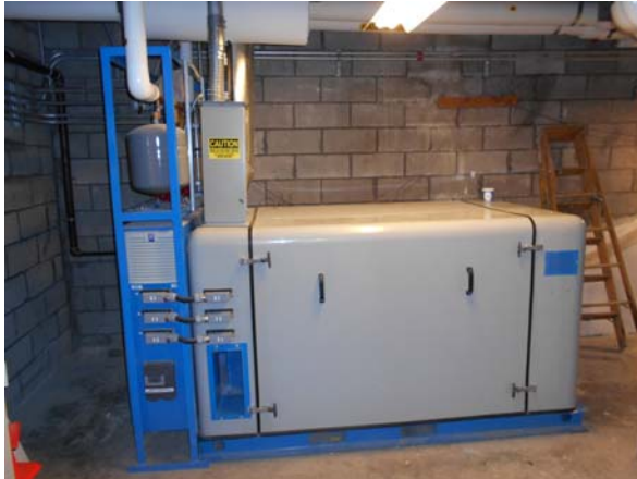
One (1) Aegen Powerverter (PV-75) cogen units located in cogen room in sub-basement level parking garage.
