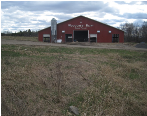
Existing Heifer Facility.
