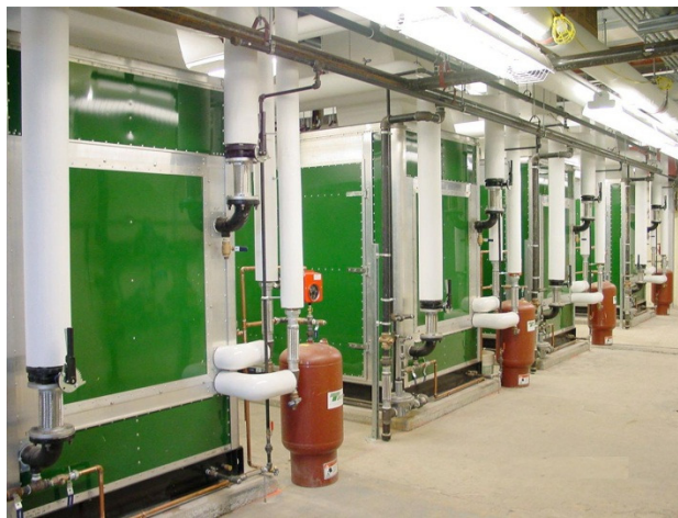
FIGURE 3 ENGINE-GENERATORS IN SOUND ATTENUATION ENCLOSURES
