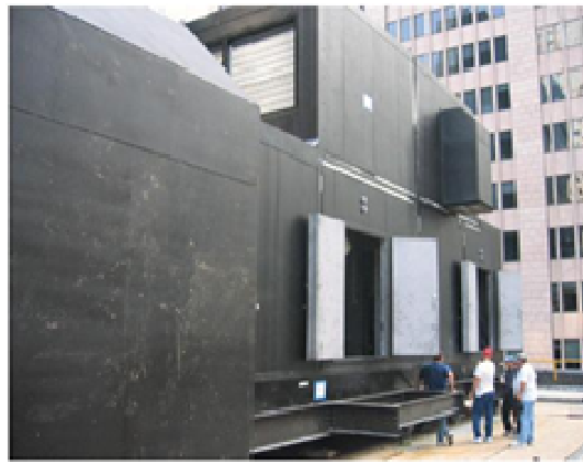
FIGURE 7 FINISHED SOUND ATTENUATION ENCLOSURE
