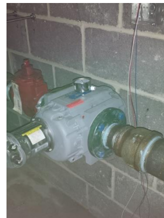
Utility Gas Meter (FG)
