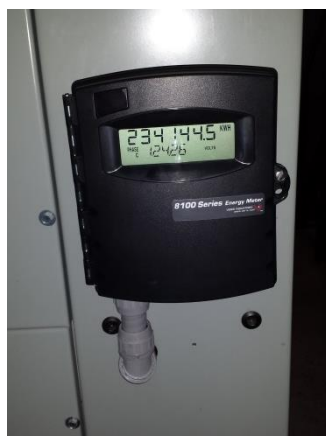
Veris 8100 Series Energy Meter (WGNet)
