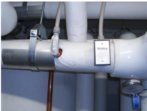
Unknown Thermistor (TLR3_Alt) and Onicon System-10 Thermistor (TLR3)
