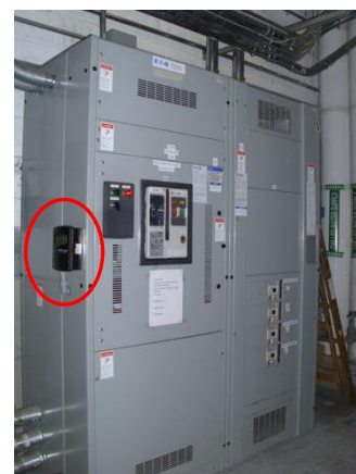
Cogen Distribution Panel (WGNet) and Veris Meter
