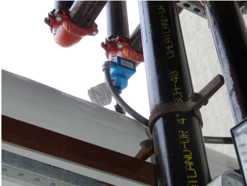
Main Hot Water Header – BTU meter
