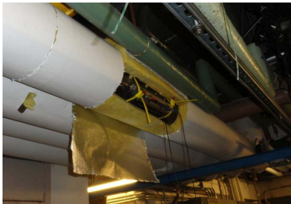
Main Hot Water Header – BTU meter
