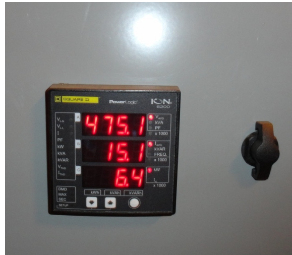
Parasitic Panel MP-1 Meter – WPAR2
