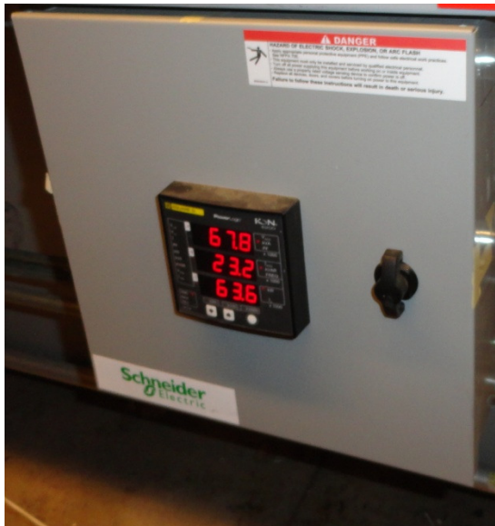
Parasitic Panel PPH Meter – WPAR1
