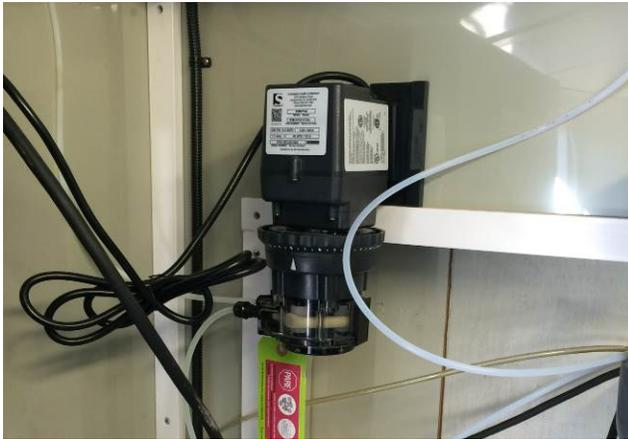
Dosing pump; injects nutrients into feedwater to bioreactor.
