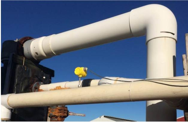
Scrubber biogas flow meter; measures biogas leaving scrubber (biogas + air injection).
