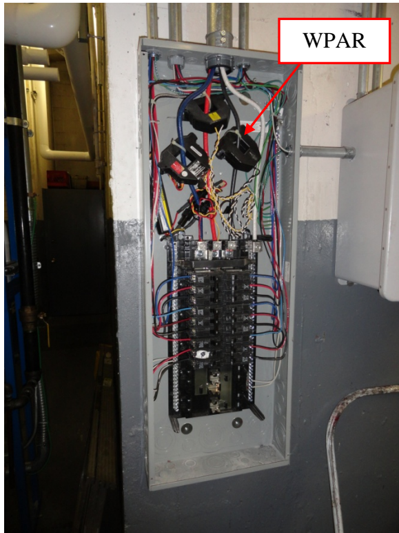
Parasitic Power Panel
